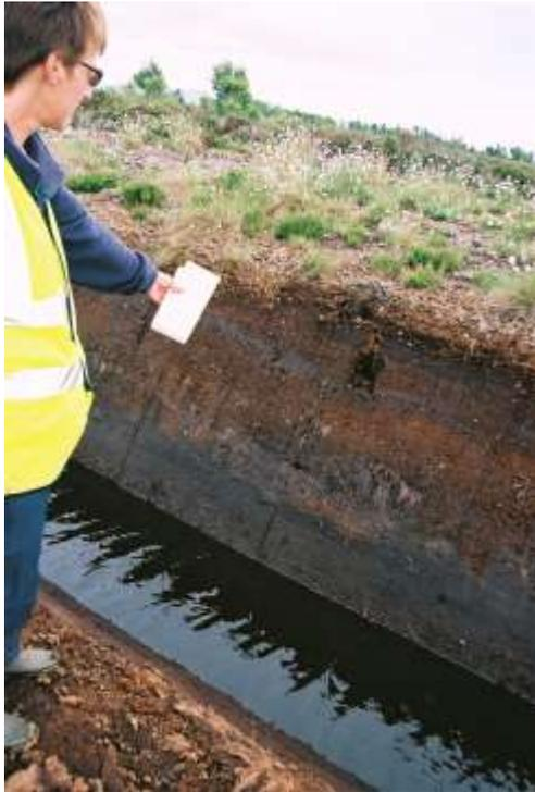
Figure 14 Drain cut in raised bog, Cumbria, to enable commercial peat extraction
