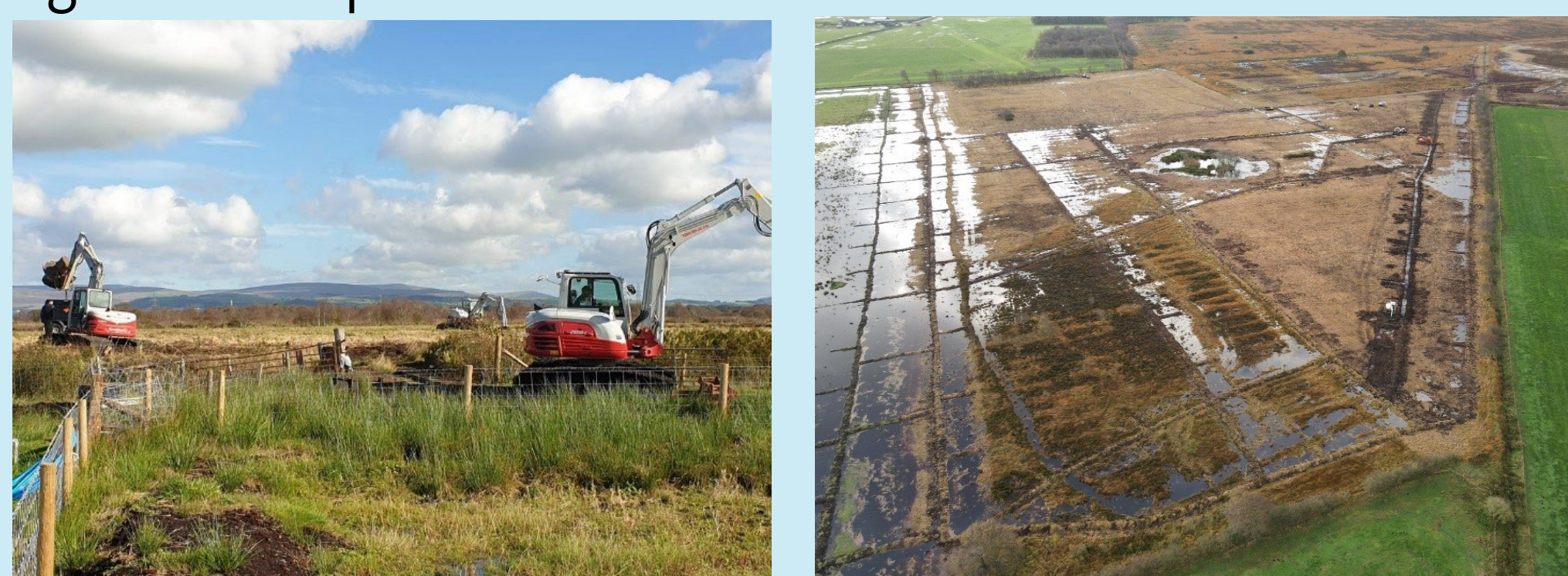
Winmarleigh Moss trench bunding and Cockerham Moss restoration. Photo credits: Lancashire Wildlife Trust
