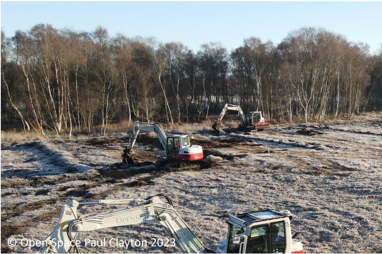
Trench bunding and tree mulching in action!
