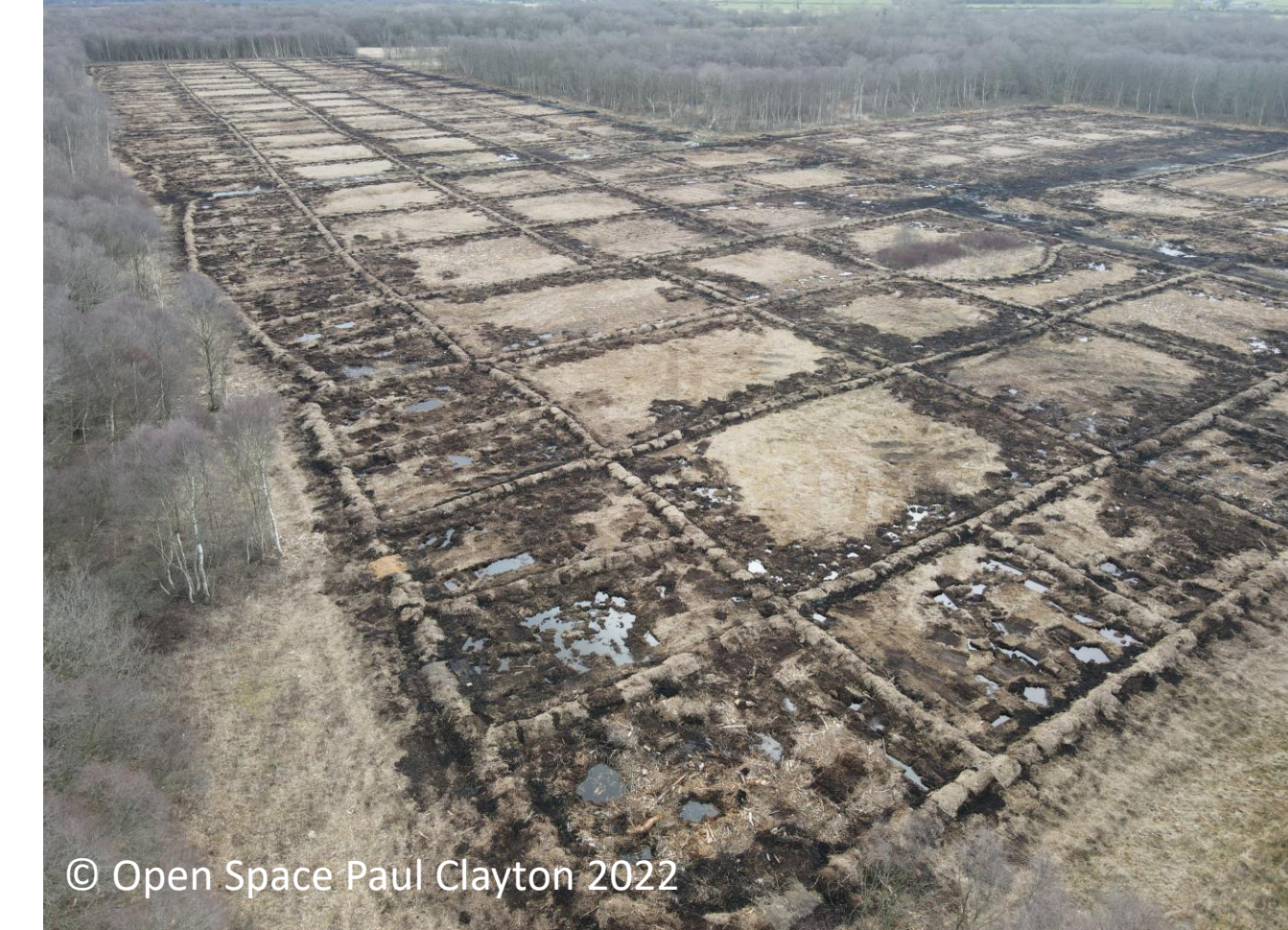
Right: Immediately after trench bunding works completed
