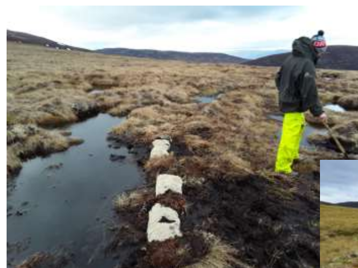
Hand-built hessian sack dams
